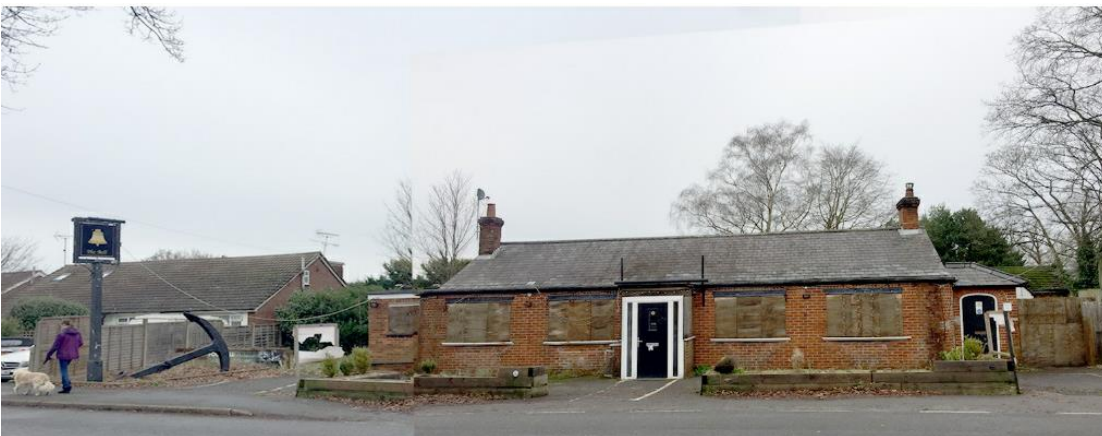
Figure 2 - Frogmore Road frontage.
